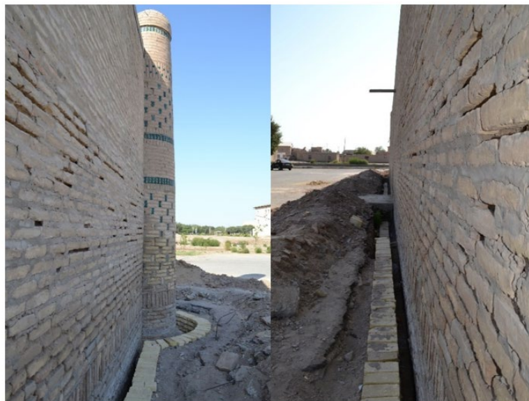
Figure 4: Application of the trench-type Khataba system on the eastern wall of the Bikajon Bika madrasa.
