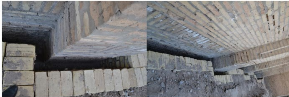
Figure 7: Application of the trench-type Khataba system on the northern and northeastern walls of the Bikajon Bika madrasa.
