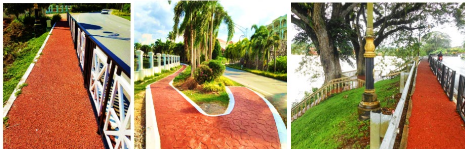
Figure 5: Permeable pavement along pedestrian paths in Zone B enhances pedestrian comfort, surface drainage, and streetscape attractiveness.
