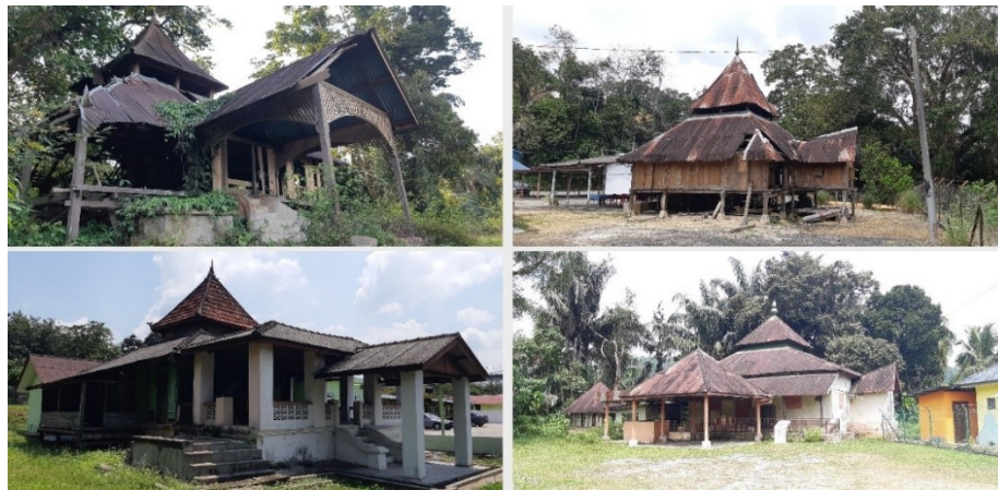
Figure 1: Dilapidated masjid in Negeri Sembilan. Masjid Lama Kg. Pelangi (Top Left), Masjid Lama Kampung Parit Istana (Top Right), Masjid Jamek Lama Tanah Data (Bottom Left), Masjid Tua Kampung Tengah (Bottom Right).
