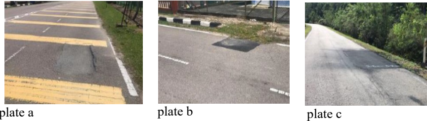
Figure 12: Patches on TRP Road (Source: Researcher's Observation)
