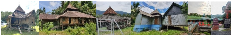
Figure 1: The dilapidated state of Masjid Lama Parit Istana, Masjid Lama Kampung Pelangai, Masjid Lama Tanah Datar, and Masjid Lama Padang Lebar.
