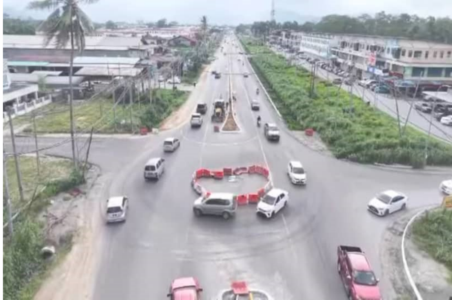
Figure 6: One of the Roundabout located in Kota Marudu Town Source: Author, 2025
