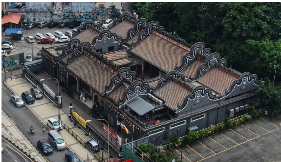
Figure 3: Aerial View of Chan She Shu Yuen Clan Shu Ancestral Hall, Kuala Lumpur, Malaysia Source: Author's Survey, 2024
