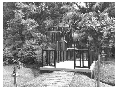
d) Platform stairs at the second entrance
