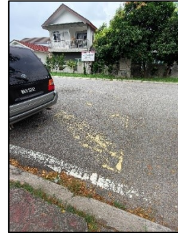
Figure 4. There are no clear markings on the speed hump
